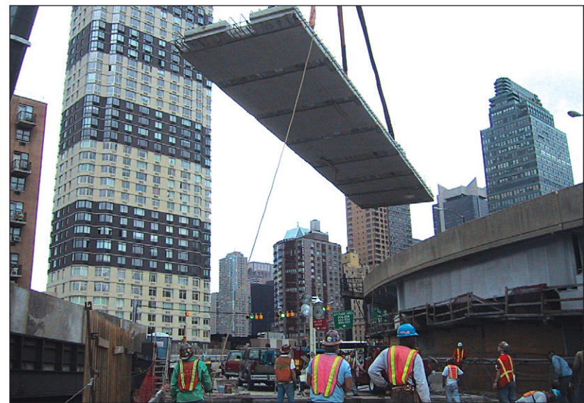
A concrete deck piece is lifted for placement.
