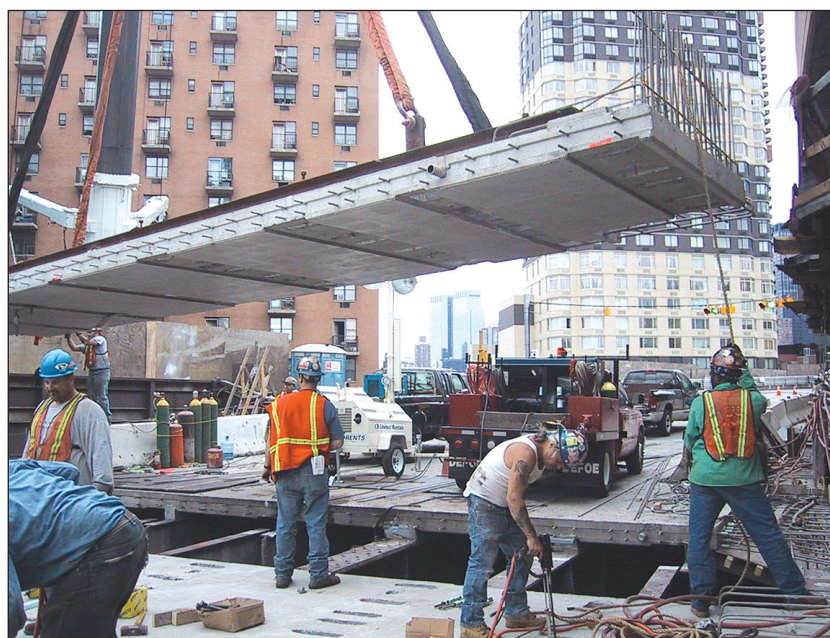
A piece of precast concrete is lowered into place.
