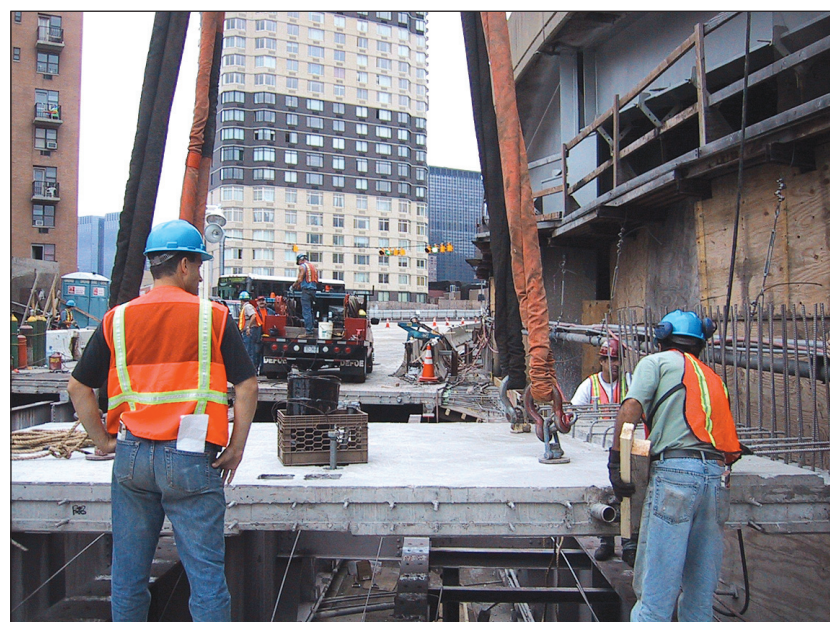
Workers prep one of 11 concrete slab replacements.
