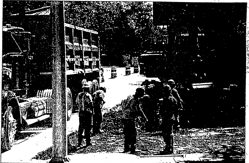
A Caterpillar hydraulic backhoe removes old concrete paving and excavates subbase for a new approach ramp to the on-grade section of Bruckner/Cross Bronx Expressway Interchange Rehabilitation Project.
